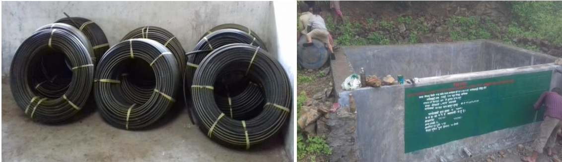
Supported Pipe & under construction RVT in Lahape, Baseni Thar
